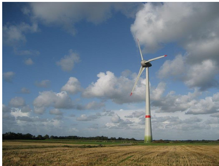
Figure 15 - Wind turbine model Enercon E-126 with rotor diameter of 126m [1]
