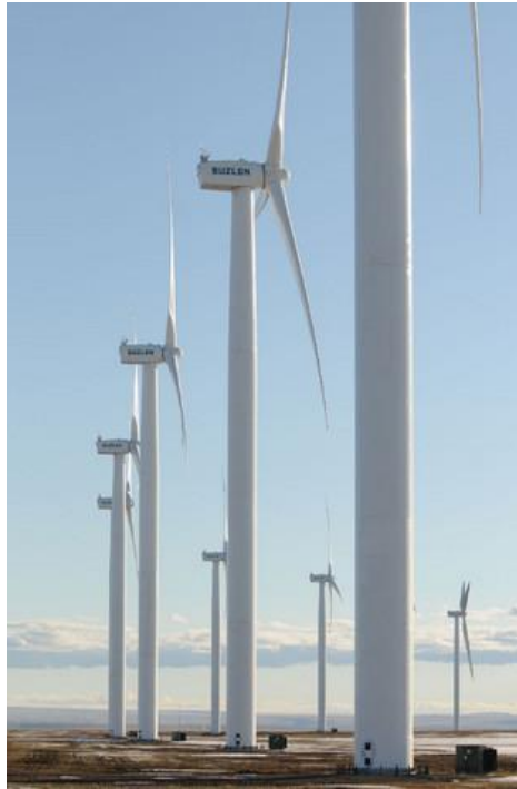
Figure 14 – Wind turbine model Suzlon s66 with rotor diameter of 66m [12]
